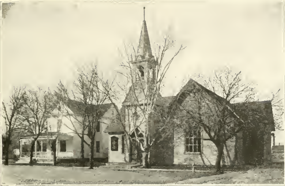
METHODIST EPISCOPAL CHURCH AND PARSONAGE, CLAY CENTER
